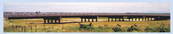
or salt-laden fogs from de-icing salts or coastal conditions are not good candidates for weathering steel. Salt precludes the development of the protective patina and dramatically accelerates corrosion.
