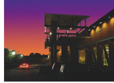
an important aspect of the look of the shops. The architect used exposed steel beams both inside and outside the buildings to preserve an industrial feel that harkens back to the site's original use. New exposed steel bow trusses were first designed for strength. However, larger sections were required by the architect to provide a more industrial appearance.
