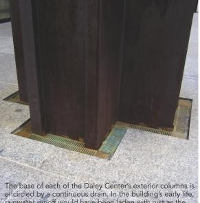
rainwater runoff would have been laden with rust as the protective patina was forming, and the drains prevented the granite plaza from becoming stained
