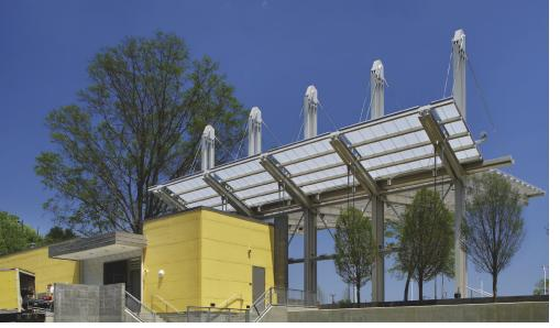
The canopy was fabricated from tapered wide-flange sections and steel tube purlins.
